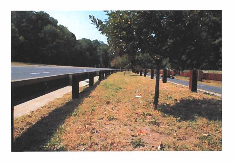
Timber Rail with Steel Plate Backing (Steel Posts or Wood Post) (TL-3)
