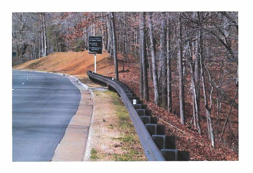
Metal Beam Rail - Powder Coated Galvanized Steel (TL-3)
