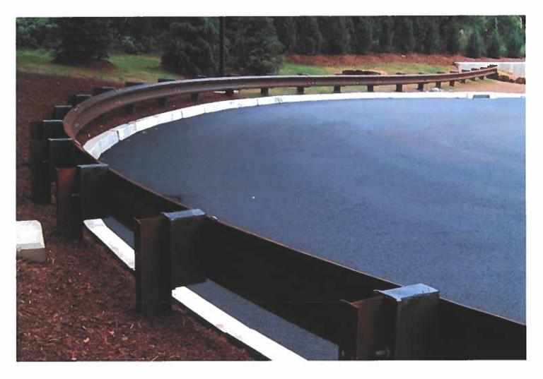
Box Beam Rail – Galvanized and Corten (Weathered Steel) (TL-3)
